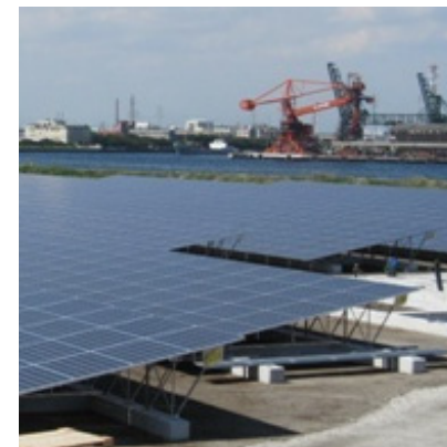
Ohgishima Solar Power Plant TEPCO
