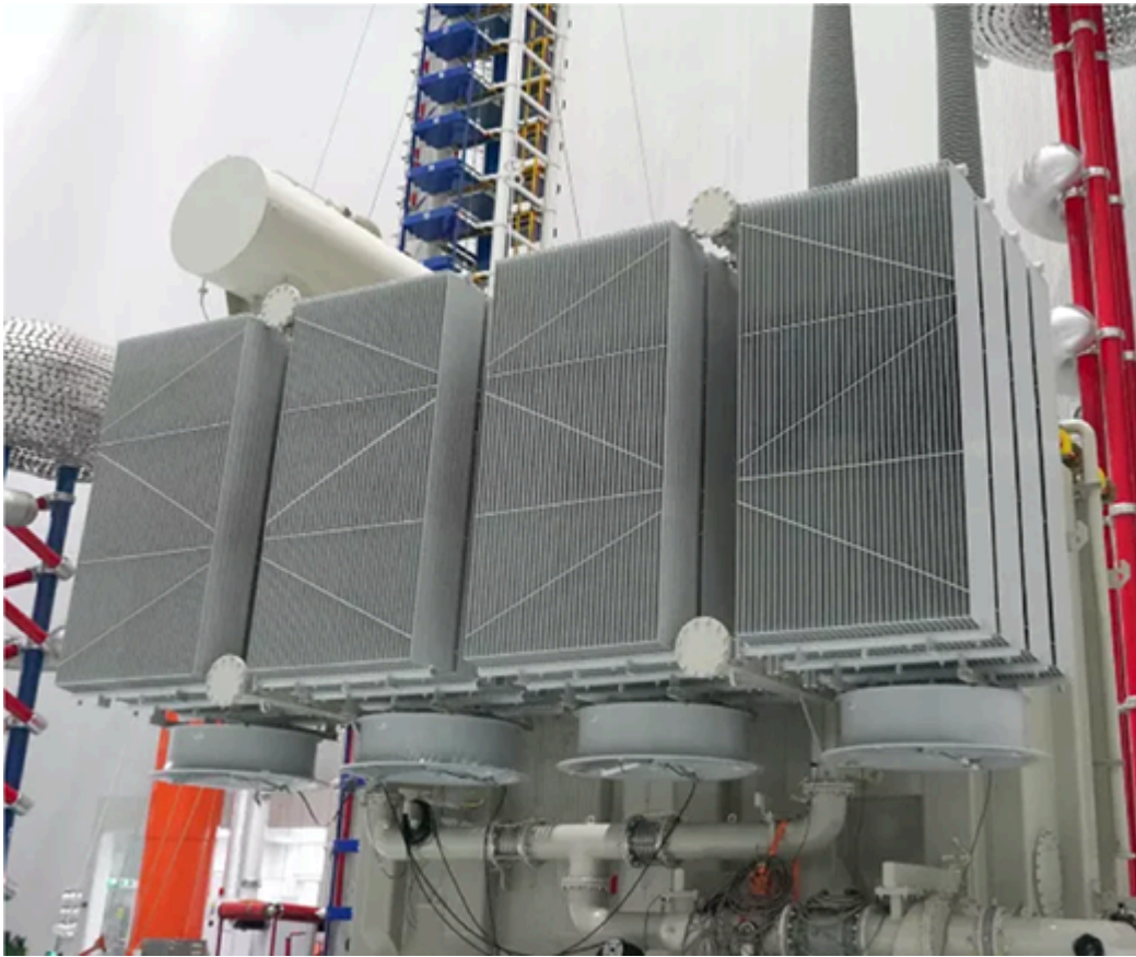
[14] World's Largest 765-kV Ester-filled Transformer
