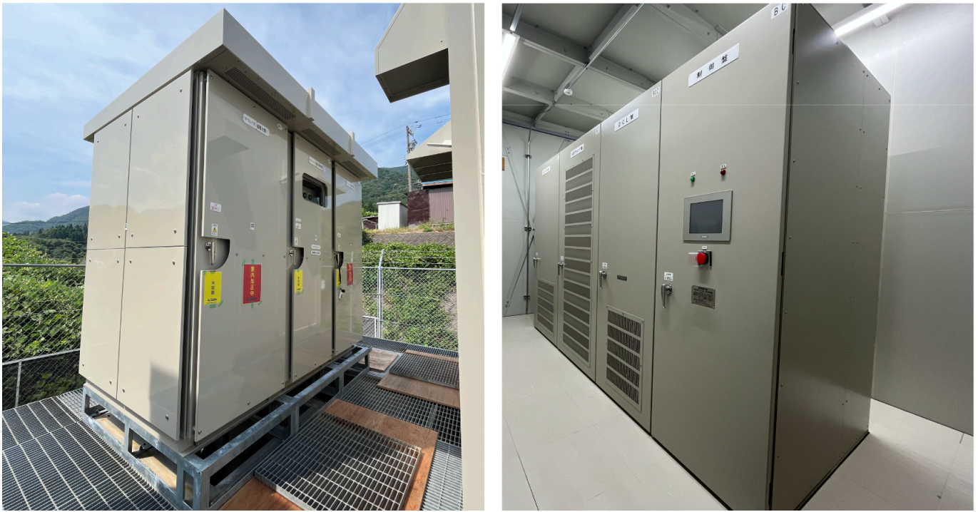
[11] B-CHOP Lithium-ion Battery Unit (left) and Converter Unit (right) Undergoing Testing
