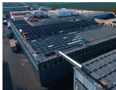
Power generation and transmission facilities, North America (image)
