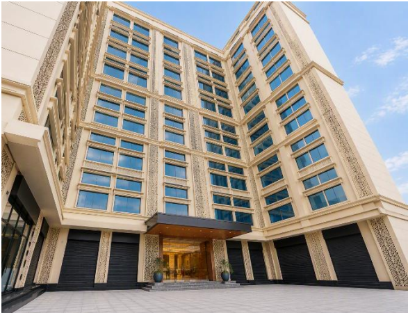
Building where the Advanced-Technology Innovation Center Mumbai (Mumbai Lab) is located
