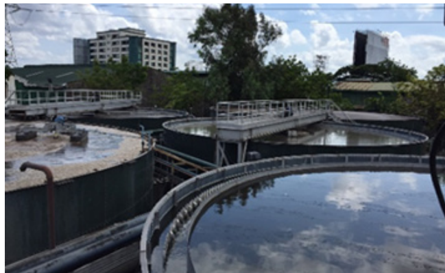
Alabang Wastewater Treatment Plant in Metro Manila
