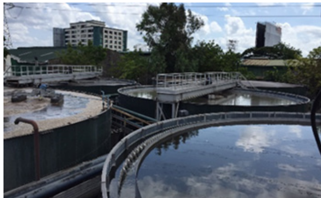
Alabang Wastewater Treatment Plant in Metro Manila
