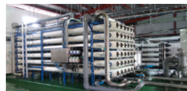
Seawater Reverse Osmosis (RO) desalination system
