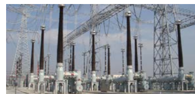
Ultra High Voltage Gas Insulated Switchgear (UHV GIS)
