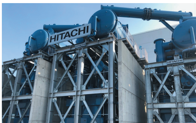
Completion of DC generator installation at the ITER Neutral Beam Test Facility (NBTF), Padua, Italy Image: National Institutes for Quantum Science and Technology (QST)
