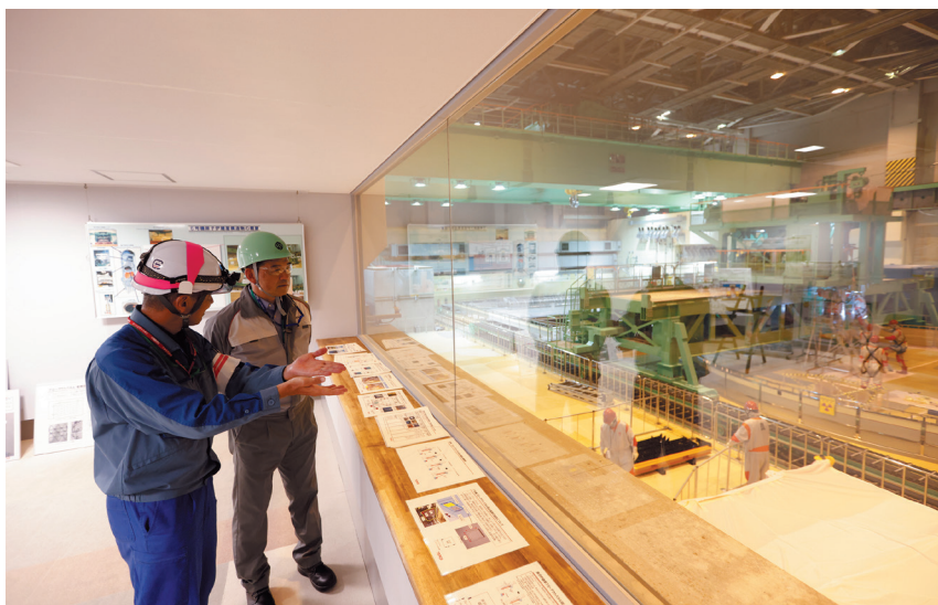
Looking out at the Unit 6 operating floor
