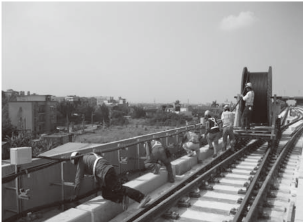
Figure 11 — Cable Laying in Progress
