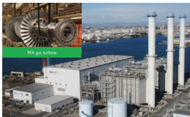
2 Advanced Gas Path (AGP) upgrade work at Ohgishima Power Station
