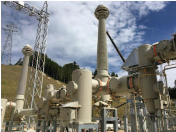
8 DC gas-insulated switchgear (DC200 kV)
