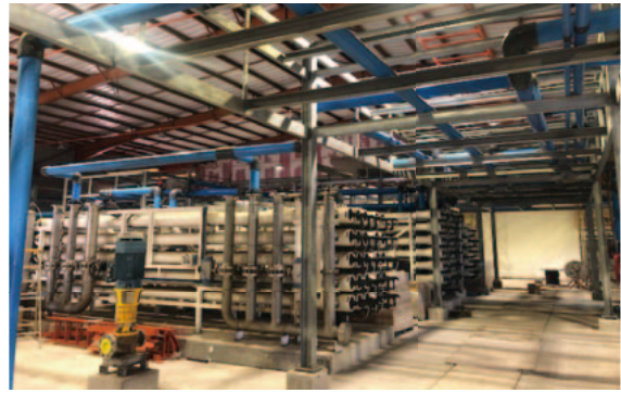
5 Integrated system of seawater desalination and sewage treatment: processing flow (left), plant under construction (right)
