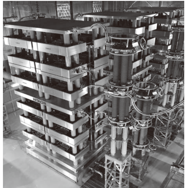
Figure 3—450-MW Thyristor Valve
