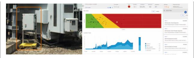
B Remote monitoring using mobile CoreSenseTM M10 (left) and diagnostic APM dashboard showing real time transformer condition
