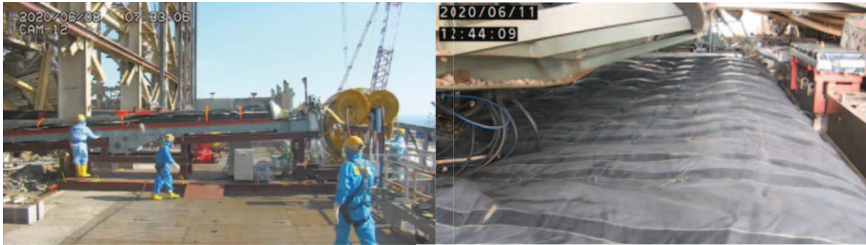
4 Checking state of SFP cover placement device (left), and SFP cover when air mortar is fully charged (right)
