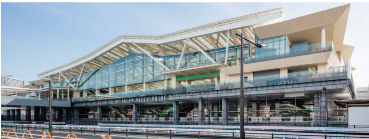
8 Building of Takanawa Gateway Station on JR Yamanote Line (photo courtesy of: JR East)
