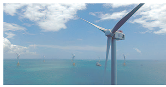
1 Taiwan offshore 5.2-MW wind turbine generators
