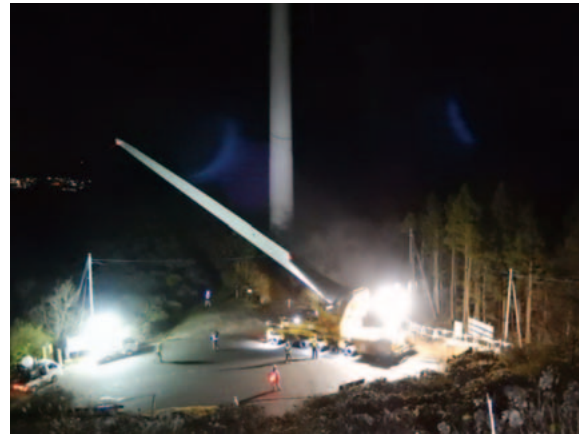
4 Operation of blade lifter
