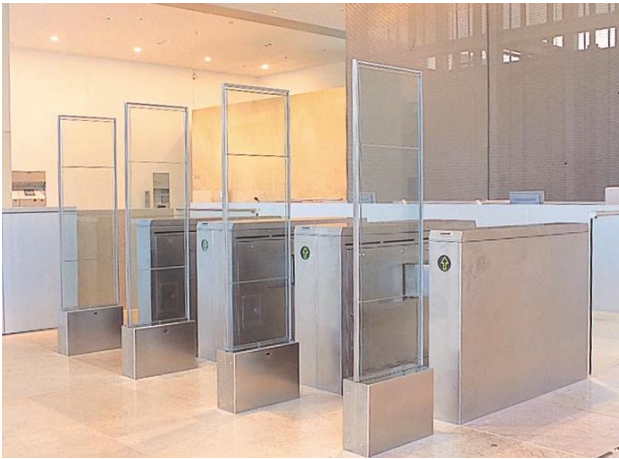
Fig. 2—Access/egress Control Gate. These gates are integrated with a function to detect tags on products to prevent shoplifting.
