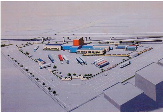
Fig. 1—Overall View of Container Inspection Center. A container inspection center is often located near a seaport container terminal. The center consists of two types of inspection facilities. One is for inspecting cargo containers using large-size X-ray equipment while loaded on trailers. The other unit is for individual inspection of all cargo inside a container when the trailer X-ray inspection identifies a suspicious piece of cargo.
