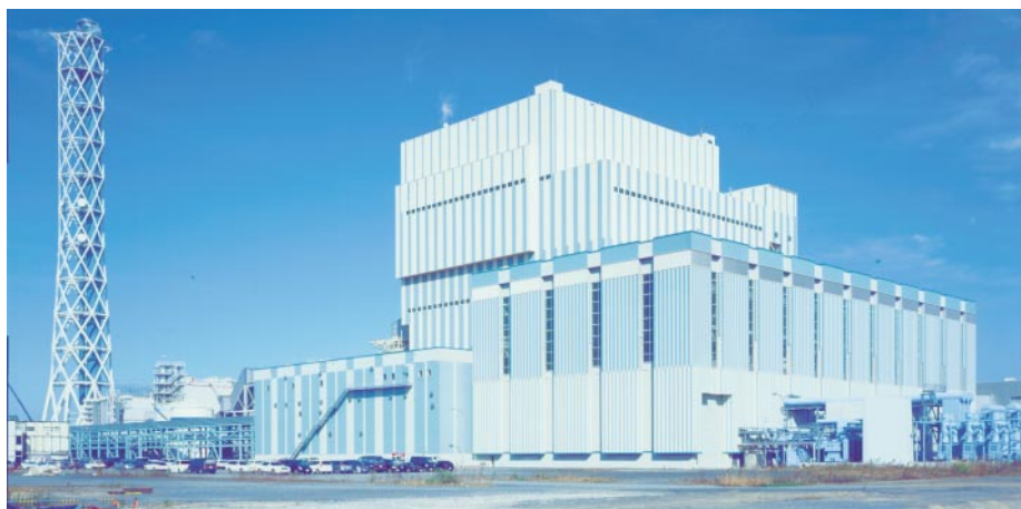
Fig. 1—View of Completed Hitachinaka Thermal Power Station. Located at Hitachinaka Thermal Power Station, Hitachinaka Port north quay Ibaraki Prefecture, Japan, Unit No. 1 — a 1,000-MW power-generation plant — was completed in December, 2003.
