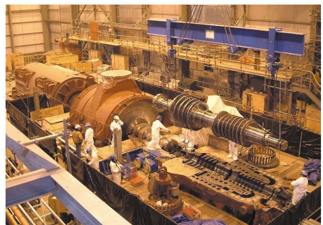
Fig. 3—Turbine Installation. High and intermediate pressure turbine rotor setting on the casing. The 40-inch-blade low-pressure turbine with inner casing and 586-MVA generator are shown behind it.
