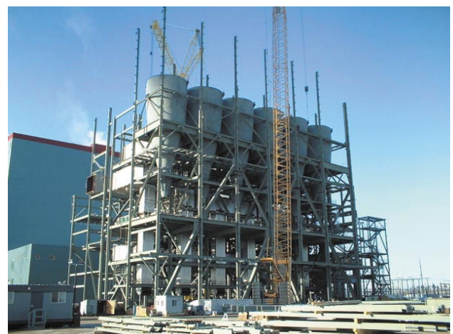
Fig. 9—Boiler Simultaneous Construction.
