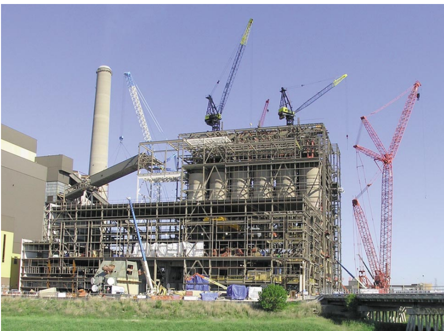
Fig. 1—Photo of Project Construction in Progress, May 2005.
