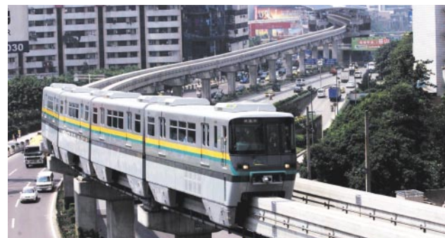
Fig. 10—Monorail in Chongqing, China. China's first urban monorail began operating on June 18, 2005.
