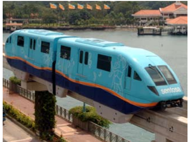
Fig. 4—Hitachi-built Sentosa Monorail. Hitachi monorail system is a cost effective urban transit that not only relieves traffic congestion but also aesthetically less intrusive and environmentally conscious.
