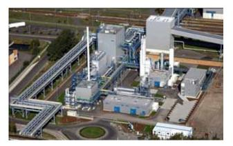
Fig. 3—Schwarze Pumpe Oxyfuel Pilot Plant. The 30-MWth class full-system oxyfuel pilot plant is operated by Vattenfall (image courtesy of Vattenfall).
