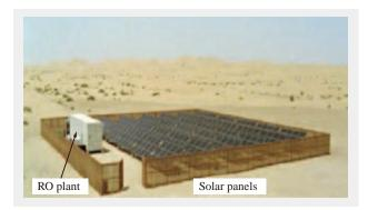
Fig. 4—Example Solar RO System Site. The 35-kW standalone photovoltaic generation system powers an RO unit which can produce 4 m<sup>3</sup>/h of fresh water.
