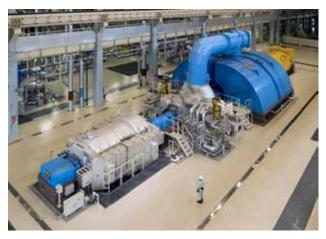
Fig. 3—New No. 2 Turbine Supplied to Isogo Thermal Power Plant of Electric Power Development Co., Ltd. The turbine operates with world-leading steam conditions, with a main steam pressure of 25 MPa, main steam temperature of 600°C, and reheat steam temperature of 620°C.
