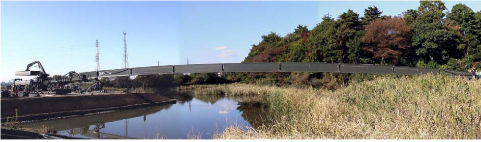
Fig. 4—Guide Beams during Deployment Process. The guide beams have a welded structure of high-strength aluminum.
