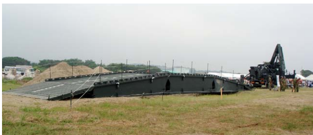
Fig. 7—Type 07 Mobility Support Bridge in Deployed Configuration.
