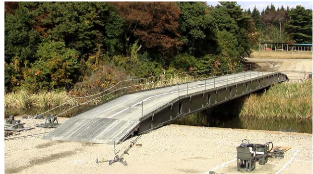
Fig. 5—Completed Bridge. The bridge sections have sufficient strength to carry heavy vehicles.
