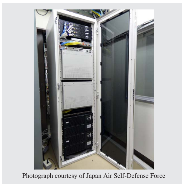
Fig. 4—Versatile Joint Communication Equipment. Exterior of main equipment for versatile joint communication installed at Matsushima Air Base of Japan Air Self-Defense Force.
