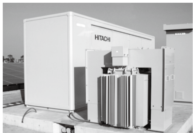
Fig. 7—Super Amorphous X ce Series Installation.
