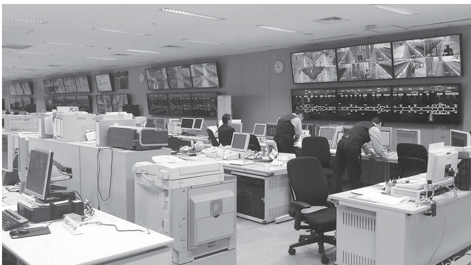
Fig. 7—Control Room at Integrated Control Center. Traffic monitoring and automatic control of all trains on four lines is handled from supervisory control desks and the traffic display panels for each line that are installed side-by-side in the control room.
