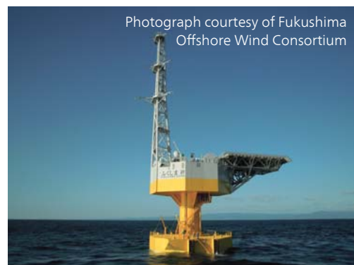
The electrical conversion equipment is installed on the top of this floating substation.
