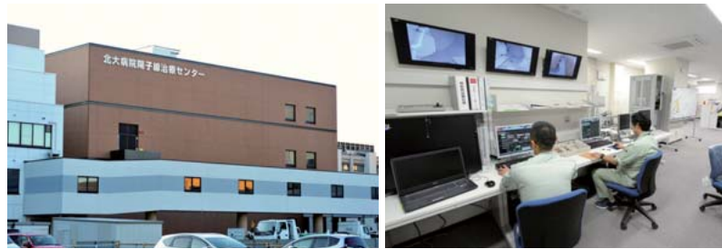
Careful adjustments are being made at the Proton Beam Therapy Center in preparation for the commencement of patient treatment.
