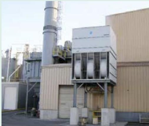
WFI's closed-loop water cooling system.
