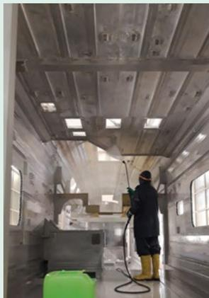
Pre-painting degreasing treatment using a VOC-free solvent.
